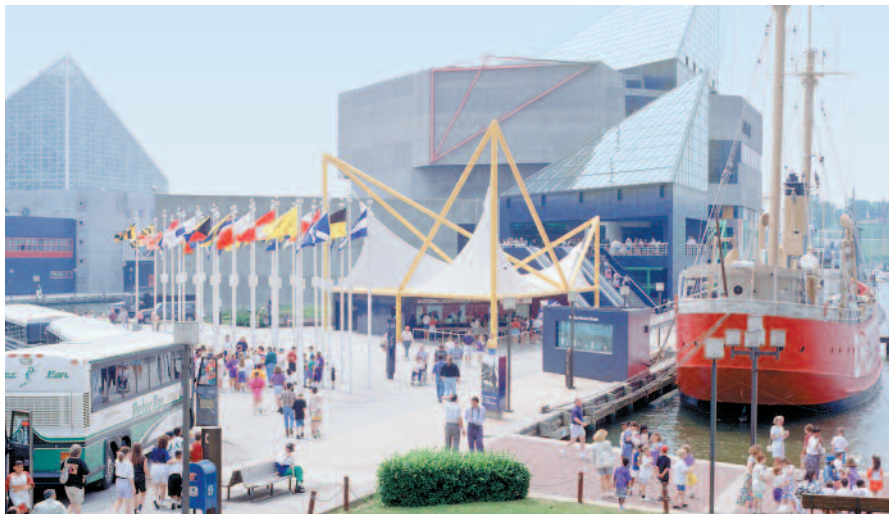
At the National Aquarium in Baltimore, Polygon helped the contractor dry out wet concrete quickly, improving adhesion and keeping the project on schedule and on budget.
