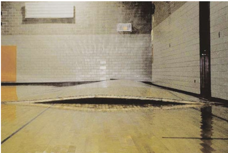
Lifting of sports floor.
