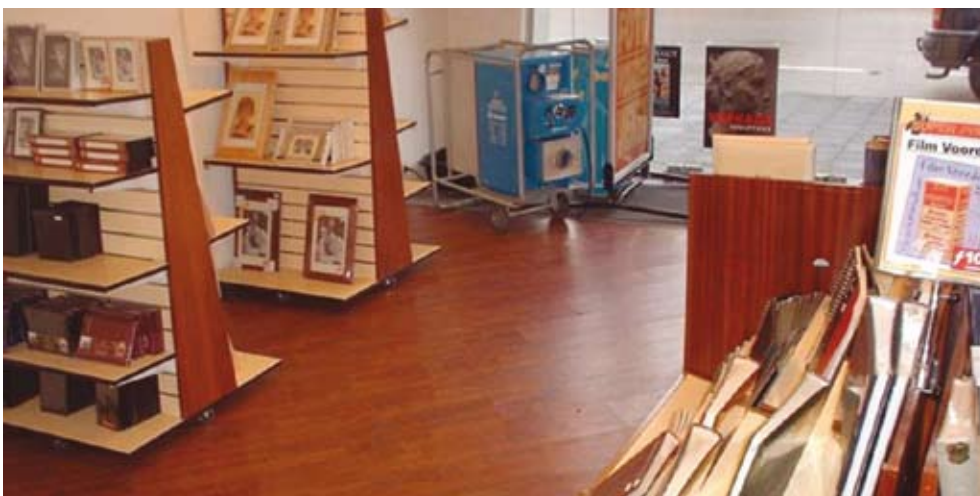
Dehumidification of damaged floor.
